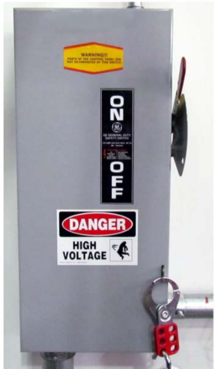
Figure 2.2 External View of 3-Phase Disconnect Panel
