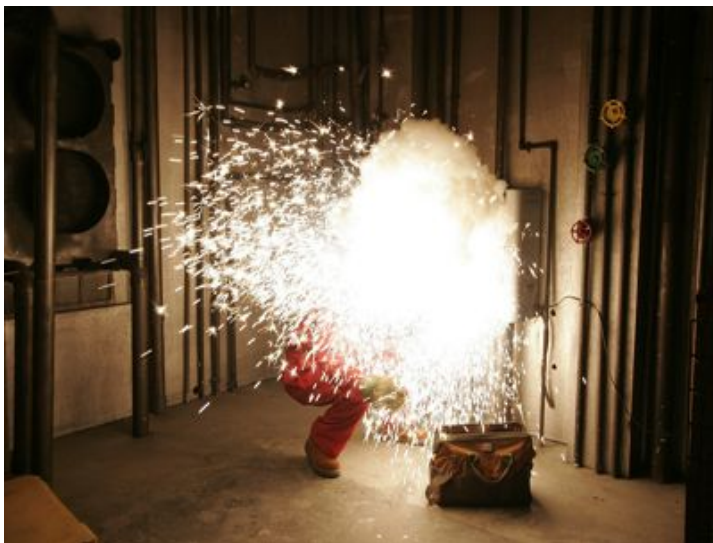
Figure 1.1 Arc Blast –©Tri-Tech Engineering
