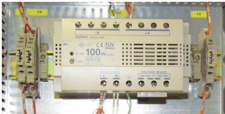
Figure 2.18 Low Voltage Power Supply
