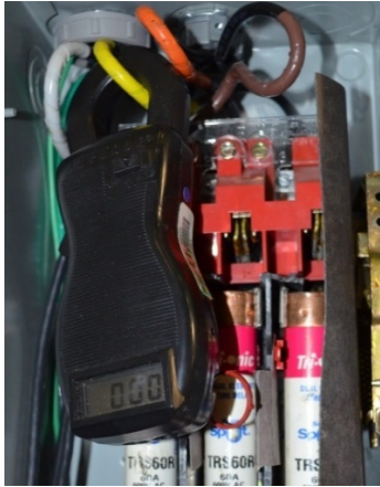
Figure 2.25 Clamp-On Ammeter
