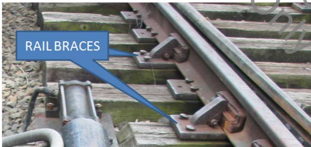
Figure 103.3 Rail Braces - Courtesy LIRR
